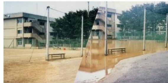
Rainwater storage at school ground
