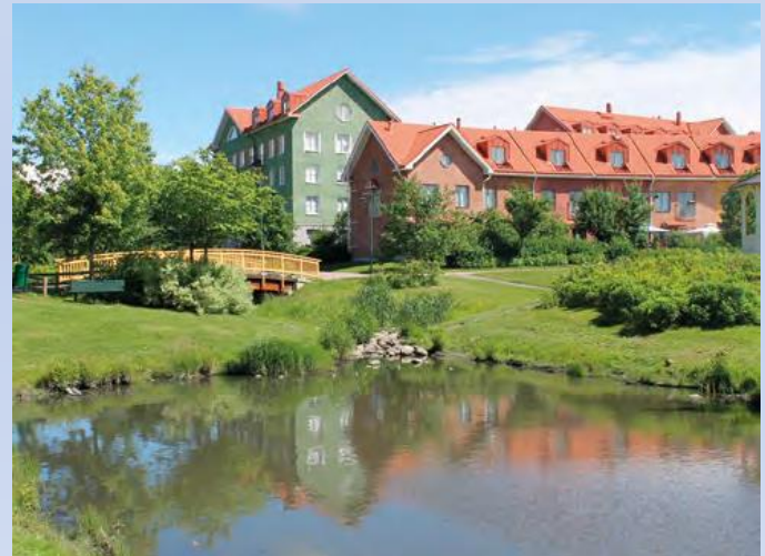
Storm water management within a residential area in Vantaa
